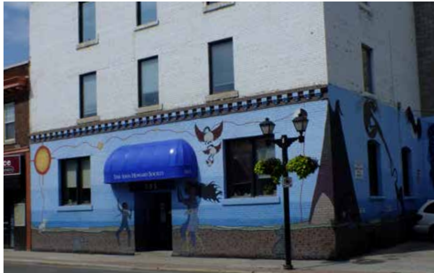
The John Howard Society of Manitoba (main floor) owns the building at 583 Ellice Avenue. Occupants include the Four Healing Roads Lodge – Community Residential Facility and the Manitoba office of the Canadian Centre for Policy Alternatives (CCPA-MB).
